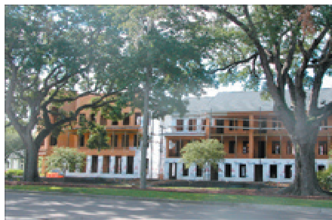
Seven Farms under construction by the Humanities Foundation will provide 72 units for families on Daniel Island.
